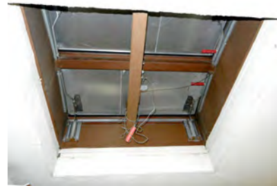
Figure 12.15. A smoke vent at the top of a stair.
