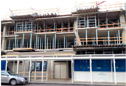
Figure 13.12. A typical 4 ft.-wide temporary walkway (painted white) over a sidewalk adjacent to a construction site. The wide span between posts accommodates the double exit doors (shown in the center), which serve an occupied cinema.
