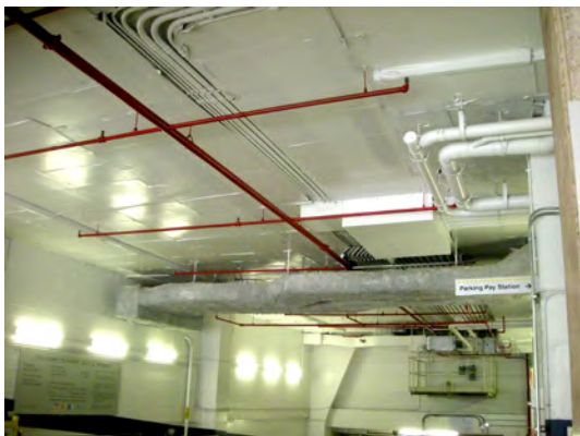
Figure 8.1. A fire sprinkler system.
