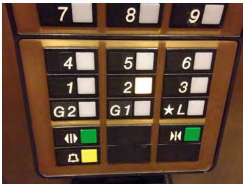
Figure 6.7. An elevator car panel in a building with both a lobby level and first floor above it.
