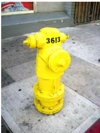
Figure 4.6. A wet barrel fire hydrant. The operating nut for the small hose outlet is on the right. The operating nut for the large outlet is on the rear of the hydrant.
