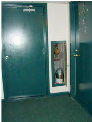
Figure 9.15. A FHC on the corridor side of a stair door (on the left).
