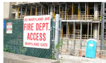
Figure 13.5. Temporary fire apparatus access.
