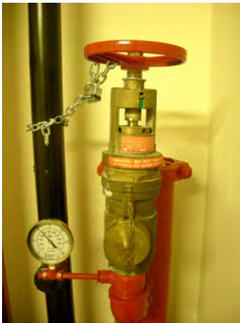
Figure 9.6. An FHC equipped with a pressure-regulating device.
