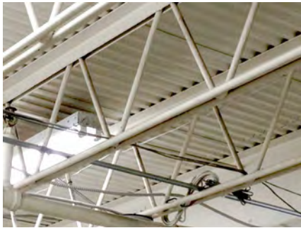
Figure 7.6. Steel bar joists.
