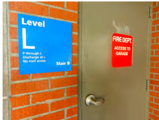
Figure 6.10. Signs outside a stair discharge door indicating fire service access (right) and the levels served by the stair (left).
