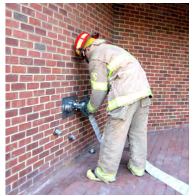
Figure 10.11. A firefighter connecting a hose line to an FDC inlet.
