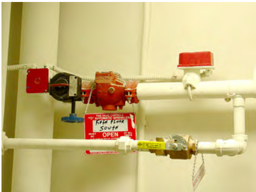
Figure 8.2. A sprinkler zone control station. The sign on the control valve indicates “first floor south” but there is no indication where the boundary is between south and north.
