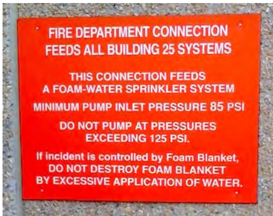
Figure 10.15. A foam-water sprinkler system FDC sign with a cautionary statement regarding the use of water.
