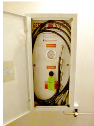
Figure 12.5. A breathing air fill panel with its door open showing air hoses.
