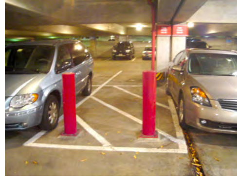
Figure 9.11. Floor striping indicates a FHC access path in a parking garage. Bollards provide vehicle impact protection. Bright signs at the top of the columns help firefighters locate the FHC.
