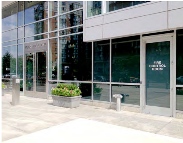
Figure 11.16. A fire command center (right) with an outside entrance next to main building entrance (left). Note the proximity of a key box (on a pedestal) and the fire department connection.
