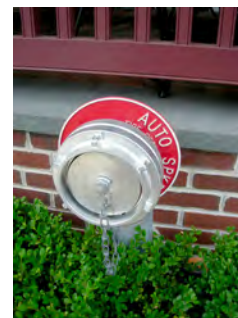
Figure 10.5. A quick-connect type of FDC.
