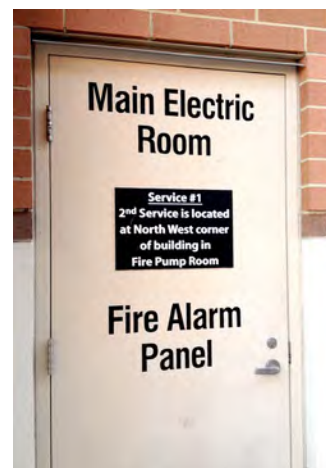
Figure 6.14. A room with signage indicating (top to bottom), the main electric service, the location of a secondary electric service, and the fire alarm system control panel.
