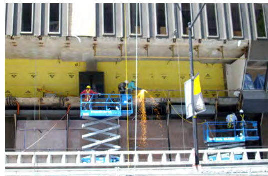
Figure 13.3. Workers on an aerial lift performing welding tasks.
