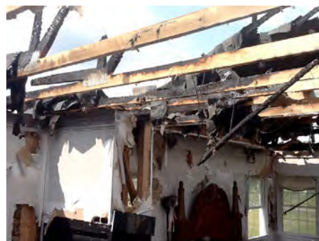
Figure 7.8. Wood trusses after an attic fire.
