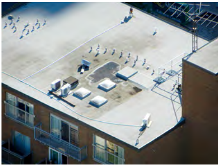
Figure 7.12. Several skylights on a roof.
