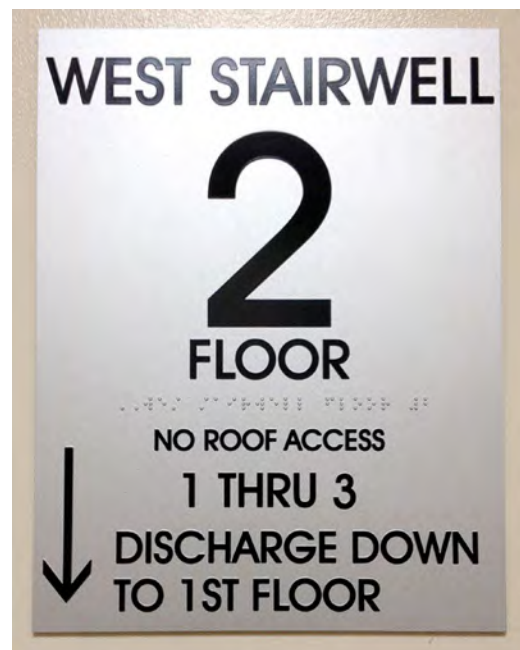
Figure 6.9. A stair identification sign.
