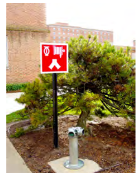
Figure 10.14. An FDC sign with the NFPA 170 symbols for both sprinkler and standpipe systems.
